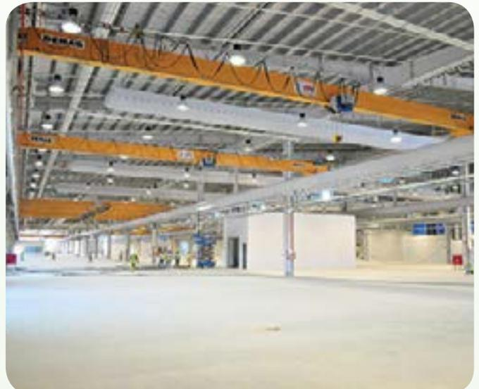
The use of fabric ducting in this factory at Tuas reduced installation times by 73%.
